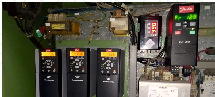
DRIVES WITH MOTOR CONVERSION
