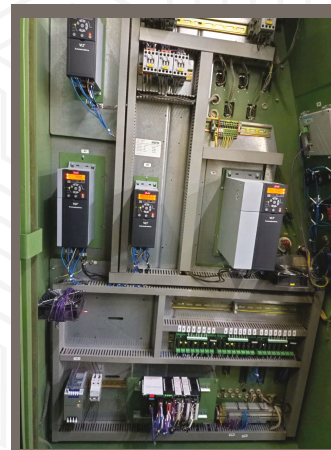
UPGRADED CARDING C50 & C51 DRIVE AND PANEL CONVERSION
